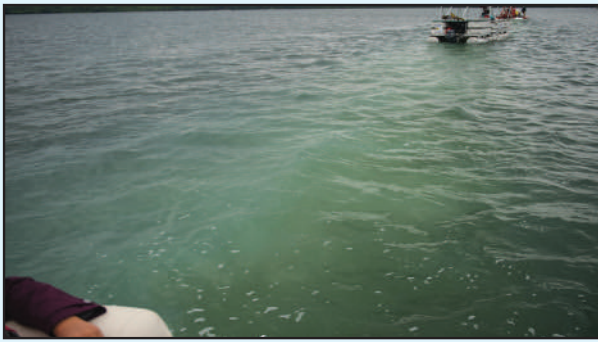
Visible alum trail behind the barge on its way into the depths to do its work
